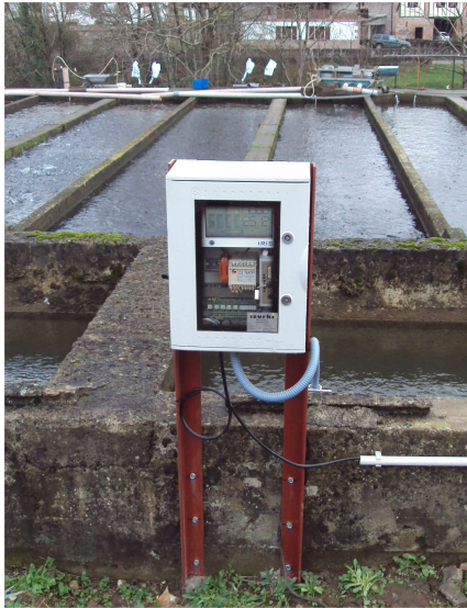
Hatchery input flow logging station.
