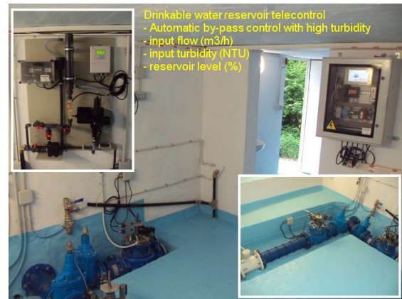
Fresh raw water reservoir telecontrol outstation.
