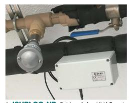
☆ î ISURLOG NB field unit for HVAC network temperatures monitoring at a health service facility.
