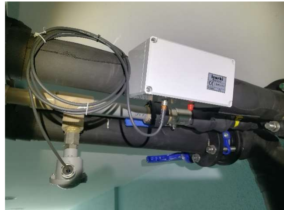
↑ Legionella prevention units in a HVAC network of a hospital, measuring supplying ring flow and temp. ⇐ IP66, 300x265x165 mm cabinet execution for robust outdoors deployment and solar panel supply.
