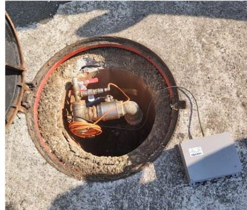
↑ ISURLOG field unit for drinkable water distribution network pressure monitoring
